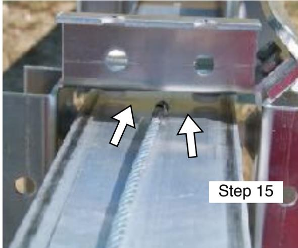
between the glide buttons and against the pole of the entire hub or the hub will not raise and lower. Let the cable lay on the ground while you complete the next step.
